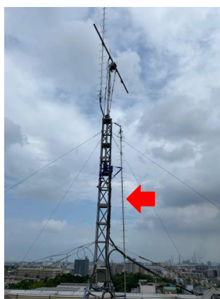
Figure 19 Antenna broken by a typhoon
